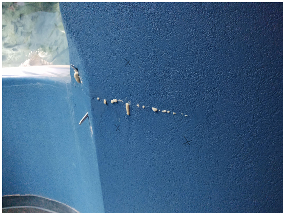
Material travel along the wall.
