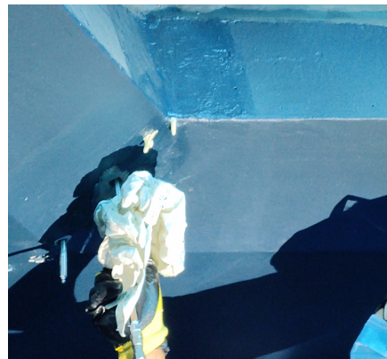
Cold Joint Injection.
