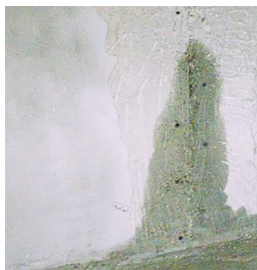
Staggered port placement on vertical crack.
